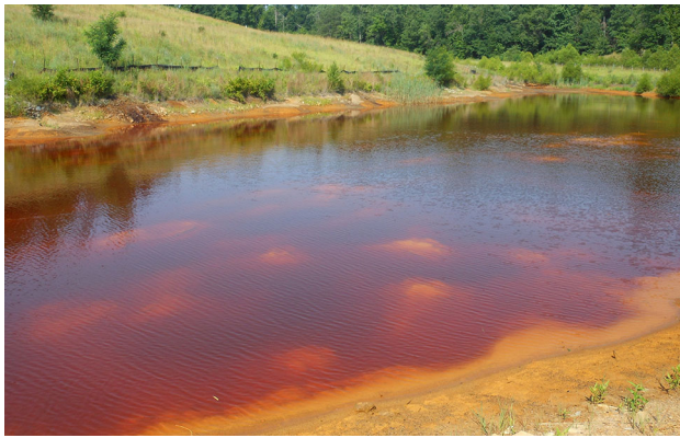
Fig. 3 The non-functional SRB filled with AMD at Tab-Simco
